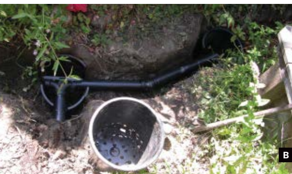
Fig. A: Black ABS pipe leads from the carport washing machine standpipe to the watering area via a trench dug under the garden path; white PVC pipe is for an unrelated irrigation system installed at the same time.
