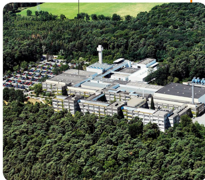
Heavy Ion Research Centre, Germany
