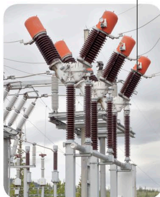
Circuit breakers
